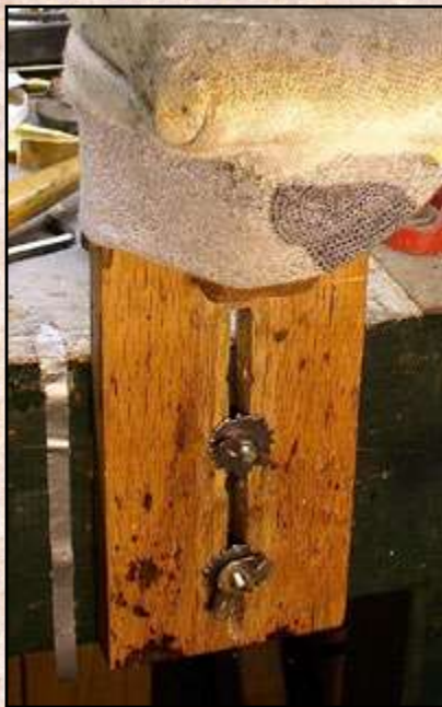
Fig. 7. I have used two means of support attachment to the fascia board. Cap bolts (1/4 x 2-12") can be inserted through the back of the board and secured with wing nuts over crenulated washers.
