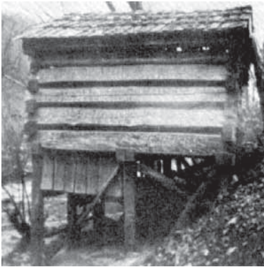
Figure 8 - After Shell's death in 1922, the remains of his grist mill on Greasy Creek were photographed. Shell learned how to build and operate a mill from his father, and after settling on Greasy Creek about 1867, he built an entire mill by himself, including all working parts, a twenty-five feet wide mill dam, and a mill race to bring water to the mill. Shell was mentally weak in his last years, but during his working life he was a capable mechanic who could do many different jobs successfully. Courtesy Leslie County Public Library, Hyden, KY.
