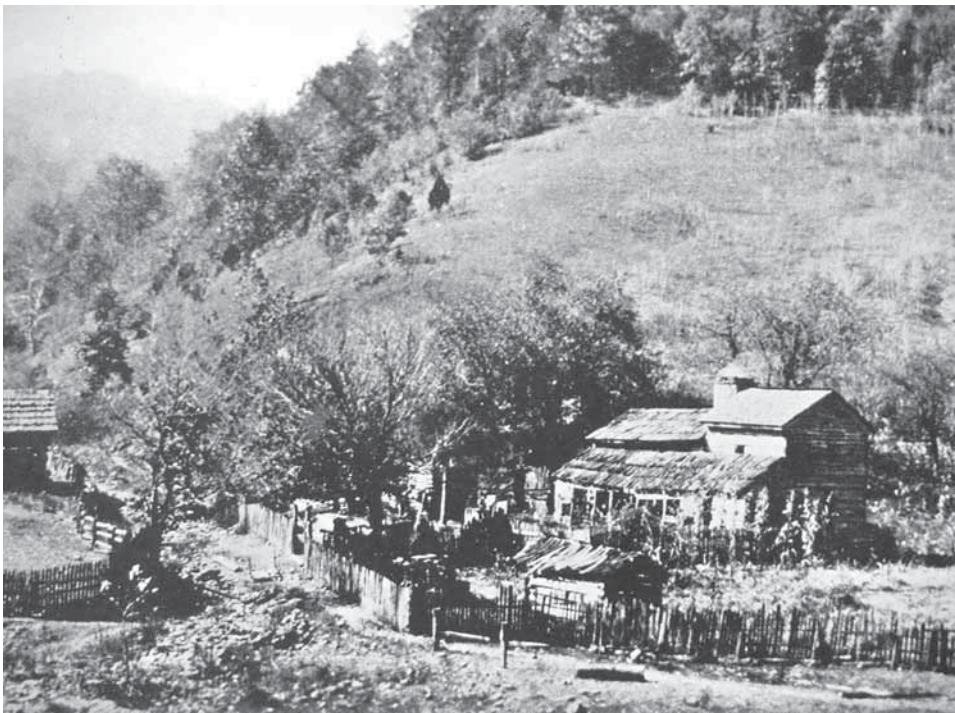
Figure 3: This early photograph of the Shell homestead was probably taken about 1900. Shell lived here for over fifty years, until his death in 1922. The extended log cabin with its center chimney and two-level roof line can be seen behind the long, lean-to style front porch. Note the hilly terrain, extensive fencing around the house and yard, the several out-buildings, and smoke rising from the chimney. The large shade trees around the house are gone today, victims of the years. From The Kentucky Rifle (1924) by Capt. John Dillin
