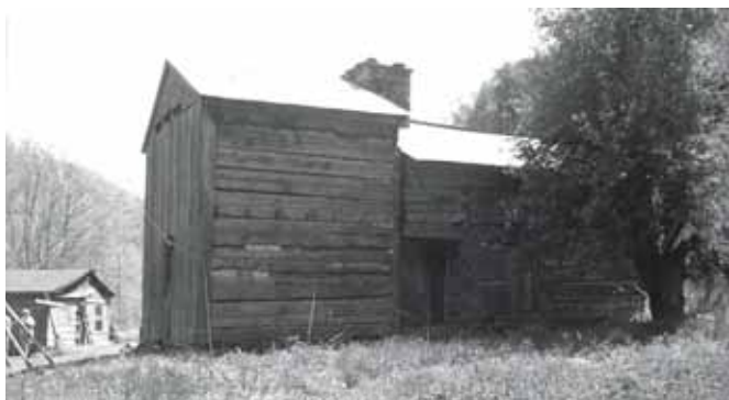
Figure 6b: The back of the Shell homestead as it appeared in 1975 clearly shows the earlier, taller cabin on the left, and the later, lower addition on the right. Both sections have an upper or second floor. Note the original clapboard siding high up under the eaves on the end of the house, indicating that the entire house was sided at one time, but over the years the siding was lost or removed. Courtesy Kentucky Heritage Council, Frankfort, Kentucky
