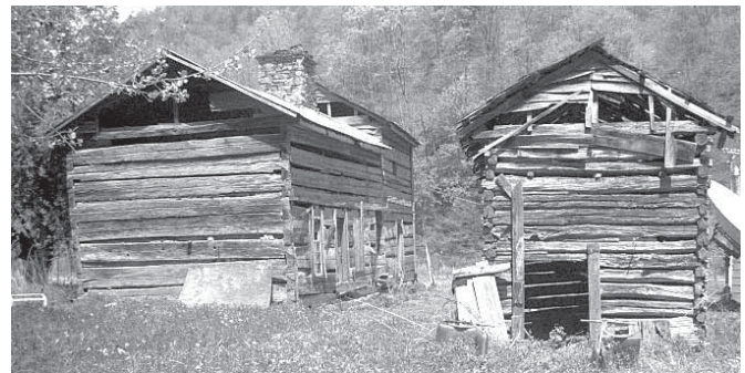
Figure 6a: This view of the Shell homestead shows the front and left end of the hewn log home as it appeared in 1975, the year it was entered into the National Register of Historic Places. Prior to that time the home had not been lived in or maintained for many years. The cabin had two front doors and a third door in the middle with stairs to the second floor. The smaller cabin to the right reportedly housed Shell's family until the larger hewn log cabin was built, but it may have simply been their smoke house. Courtesy Kentucky Heritage Council, Frankfort, Kentucky
