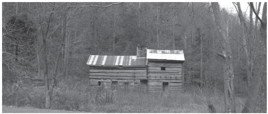
Figure 20: This is how John Shell's house looks today. It has reclaimed some of its dignity after being put on the National Register of Historical Places in 1975, and has been protected with the addition of a metal roof over the old shingled roof. The house is nestled against a hill at the end of a valley, and Greasy Creek lies off to the right. Note the original small cabin or smoke house to the left of the bigger house has lost its roof since it was photographed in 1975. Courtesy Kentucky Heritage Council, Frankfort, KY; photo by P. Kennedy.
